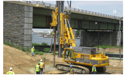
11th Street Bridge Washington, D.C.
